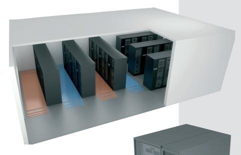
**Closed Loop:** this configuration is suitable for both "self contained" data centre and high density racks. Heat generated by server remains inside the cabinet and is disposed without entering the room.
